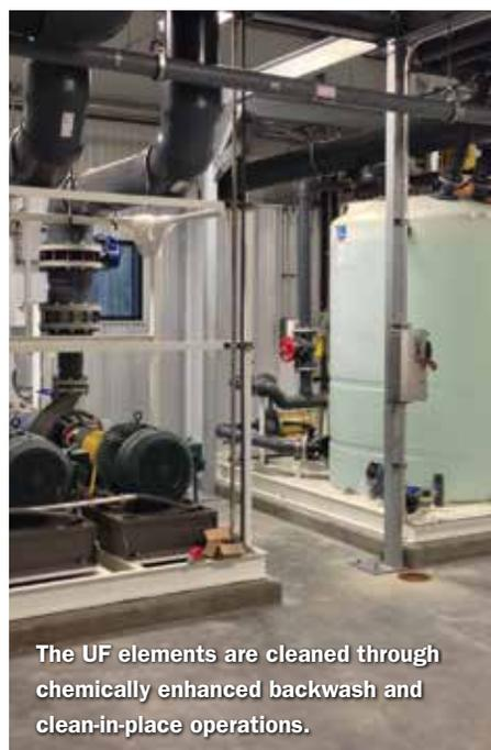
The UF elements are cleaned through chemically enhanced backwash and clean-in-place operations.
