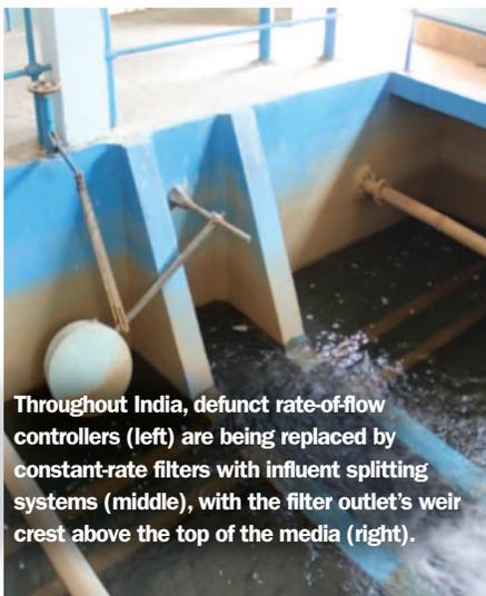
Throughout India, defunct rate-of-flow controllers (left) are being replaced by constant-rate filters with influent splitting systems (middle), with the filter outlet's weir crest above the top of the media (right).
