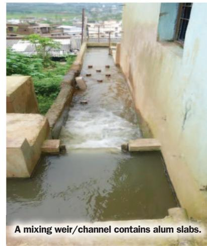
A mixing weir/channel contains alum slabs.
