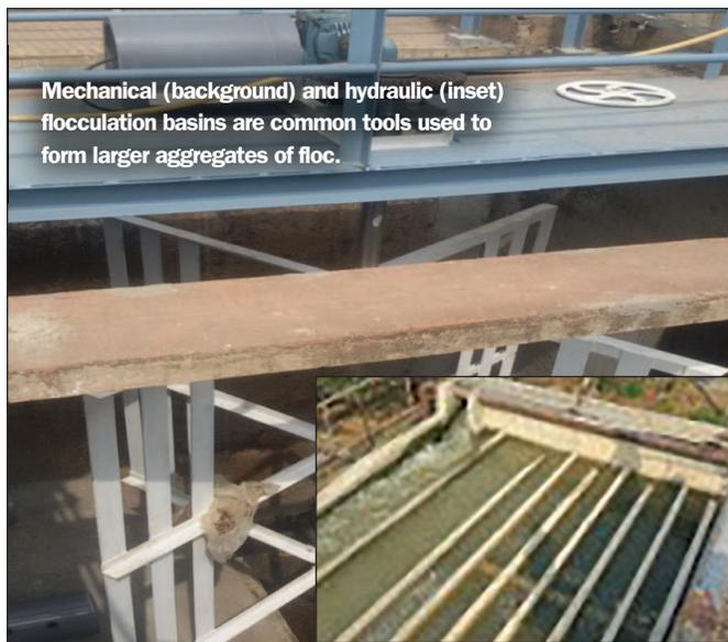
Mechanical (background) and hydraulic (inset) flocculation basins are common tools used to form larger aggregates of floc.
