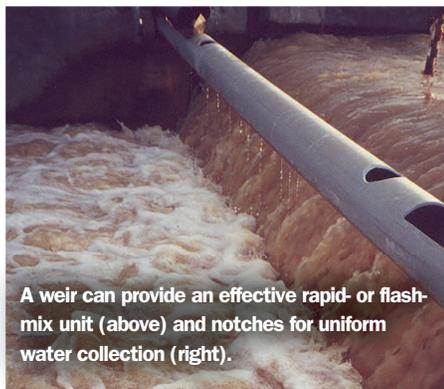
A weir can provide an effective rapid- or flash-mix unit (above) and notches for uniform water collection (right).
