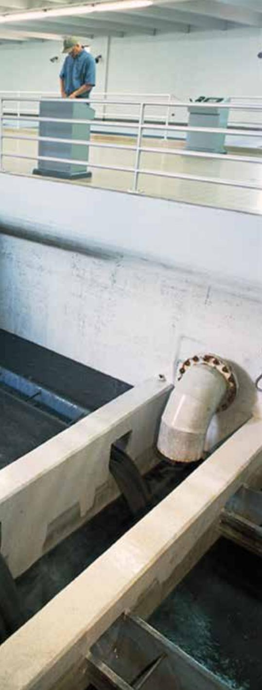
the underdrain will result in areas of high water velocity. The replacement underdrain system should be able to compensate for areas of high entrance and channel velocities to prevent lower backwash rates in these areas.
