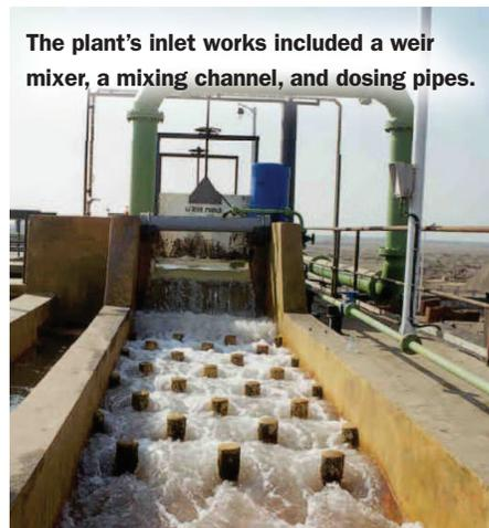
The plant's inlet works included a weir mixer, a mixing channel, and dosing pipes.
