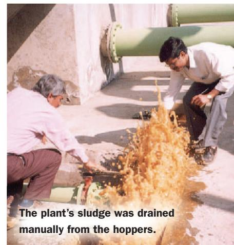
The plant's sludge was drained manually from the hoppers.
