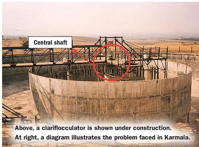
Above, a clariflocculator is shown under construction. At right, a diagram illustrates the problem faced in Karmala.
