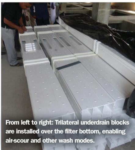
From left to right: Trilateral underdrain blocks are installed over the filter bottom, enabling air-scour and other wash modes.
